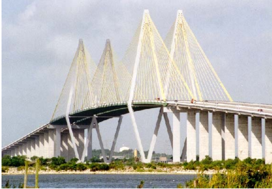
Figure 2.1: Cable Stayed Bridge (Fred Hartman Bridge at Houston, TX)
