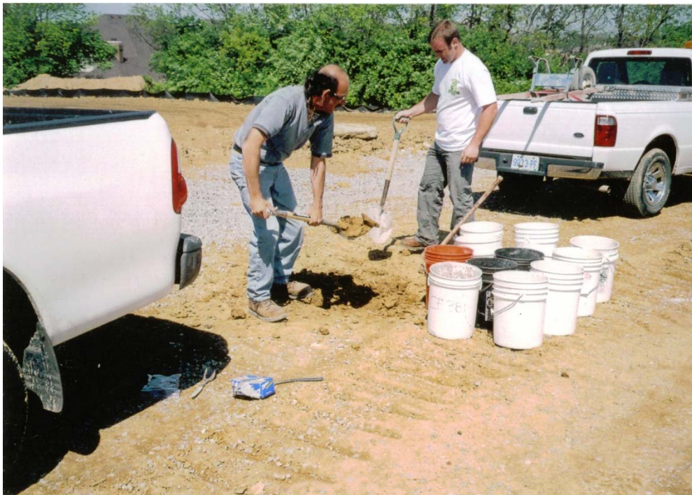
Figure 5.3 Soil Excavation Process.
