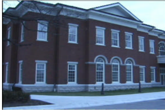
Figure 7. Building demonstrating parallel facade structure in the form of windows, trim, and face boundaries.
