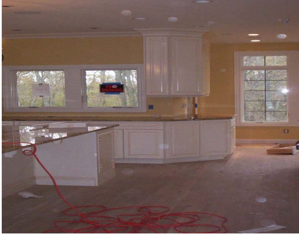
Figure B: Onsite picture 2
