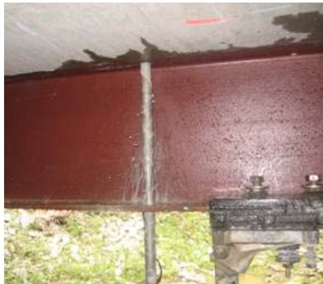
Fig. 5.8: Drilling through the bottom flange into the concrete deck
