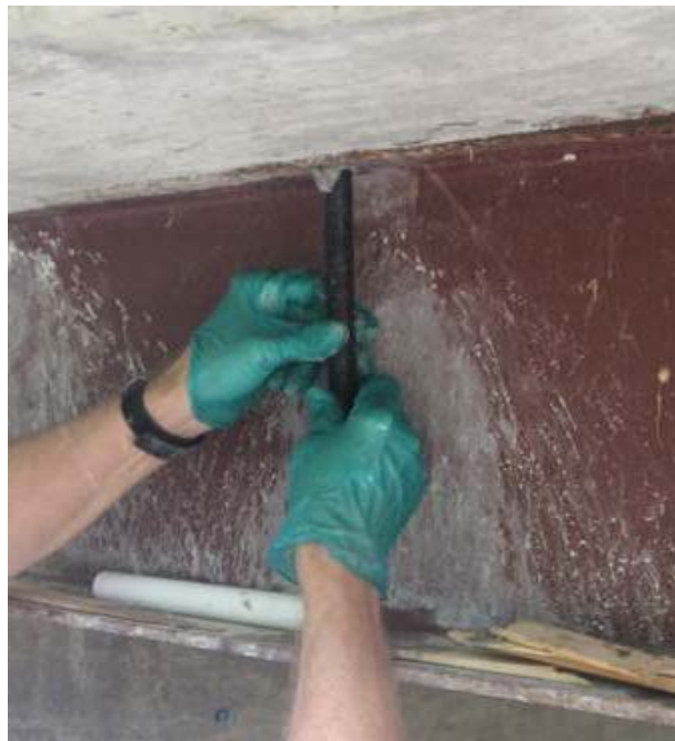
Fig. 5.10: Inserting threaded rod with twisting motion
