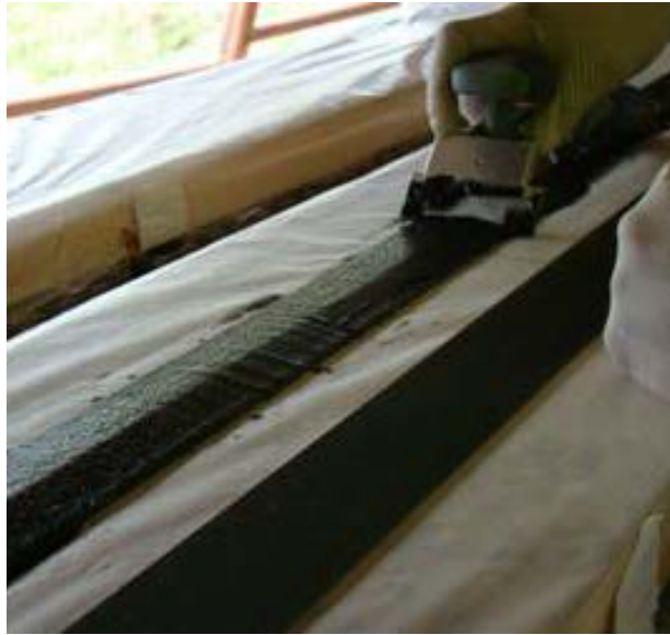
Fig. 5.19: Spreading of epoxy with V-notch trowel
