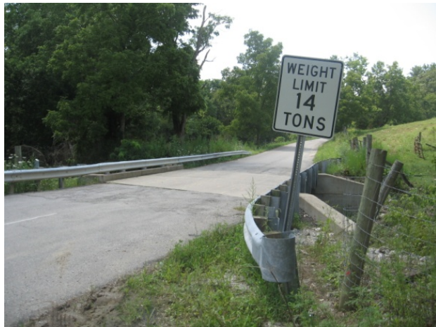
(b) View from roadway
