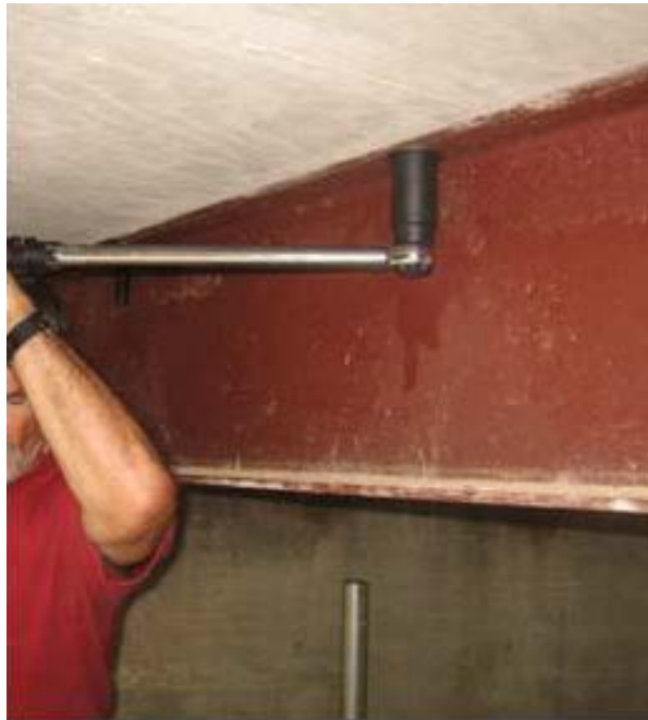
Fig. 5.12: Tightening of nut to specified torque
