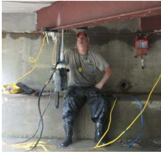
Fig. 5.7: Drilling rig fixed to the bottom flange
