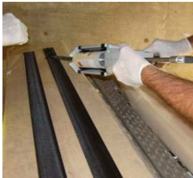
Fig. 5.18: Application of epoxy on to the top surface of the laminate
