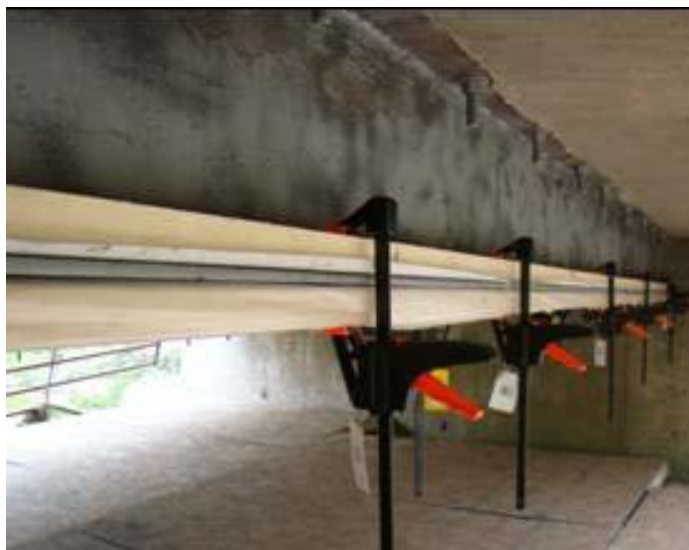
Fig. 5.21: Clamping both top and bottom laminates
