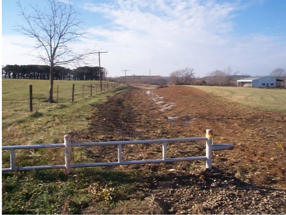
Figure 5.3: Abandoned PAL line west of Greenville, already sold off and the railbed salvaged for its gravel.
