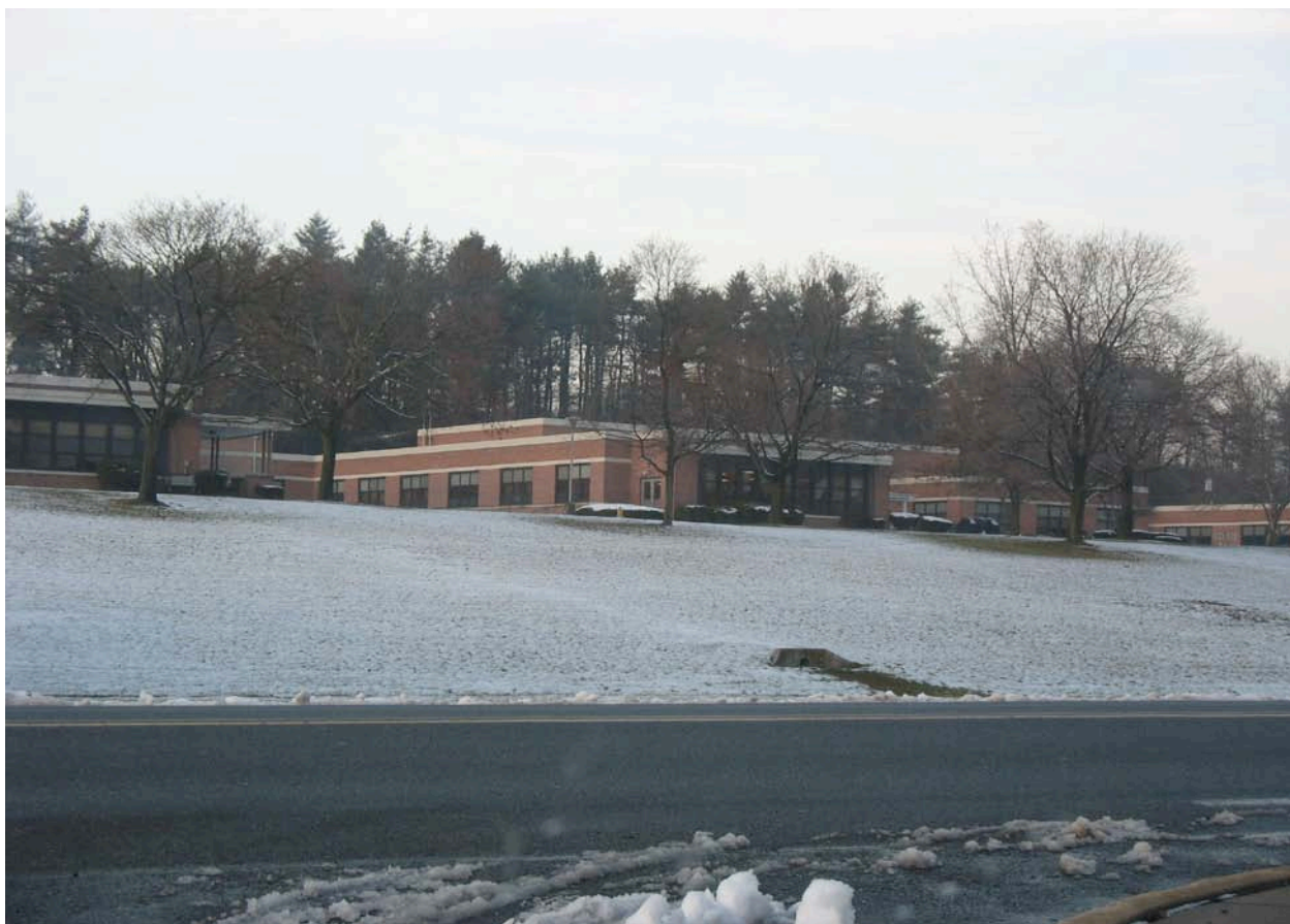
Figure 1.1: Berks County Family Shelter Care Center.
