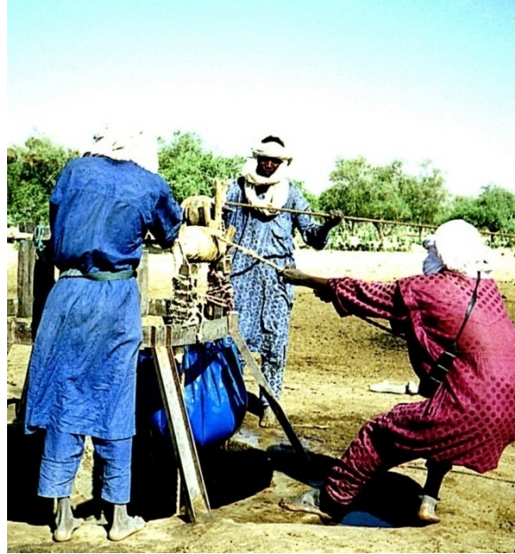
Figure 8.24: (Photo, above left, dabbunde 2003) A young Boḡaaḡo lashes forked branches and the pulley axle to the broken metal sigitahi of a large public well.
