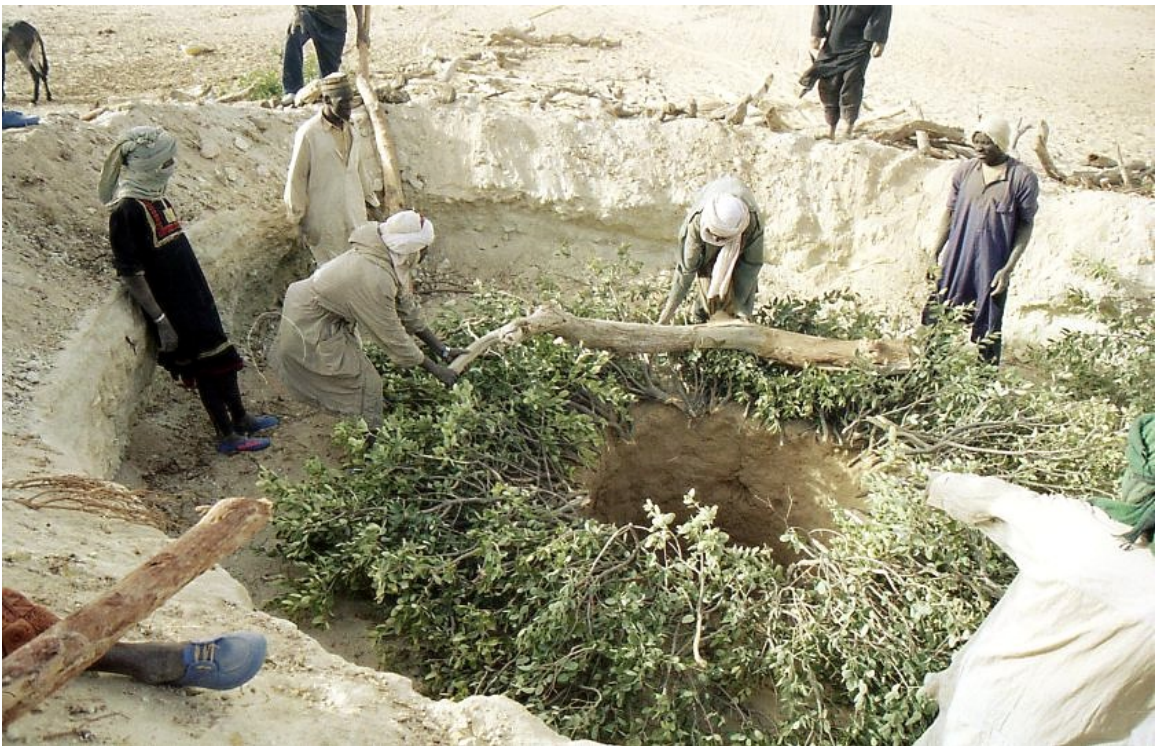
Figure 8.36: After removing all the old wood from the well mouth, the men cushion the new supports with green hanzahi branches.
