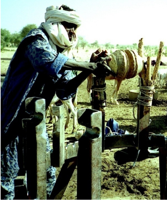
Figure 8.24: (Photo, above left, dabbunde 2003) A young Boḡaaḡo lashes forked branches and the pulley axle to the broken metal sigitahi of a large public well.
