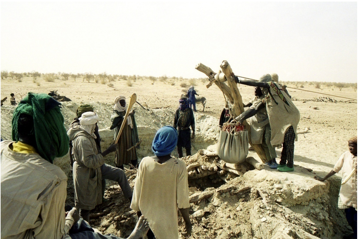
Figure 8.35: (Photo, January 2007) As they prepare to repair it, Katsinen-ko'en men dig away the earth from the mouth of Mawa well while young men pull water to empty the well.
