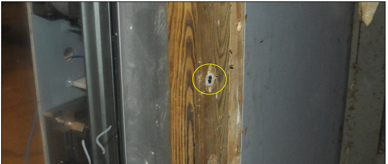
Figure 4.15 Flush Mount Sensor within Trim
