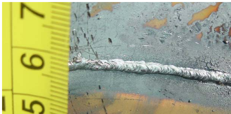
(b) Inside of the welded line
