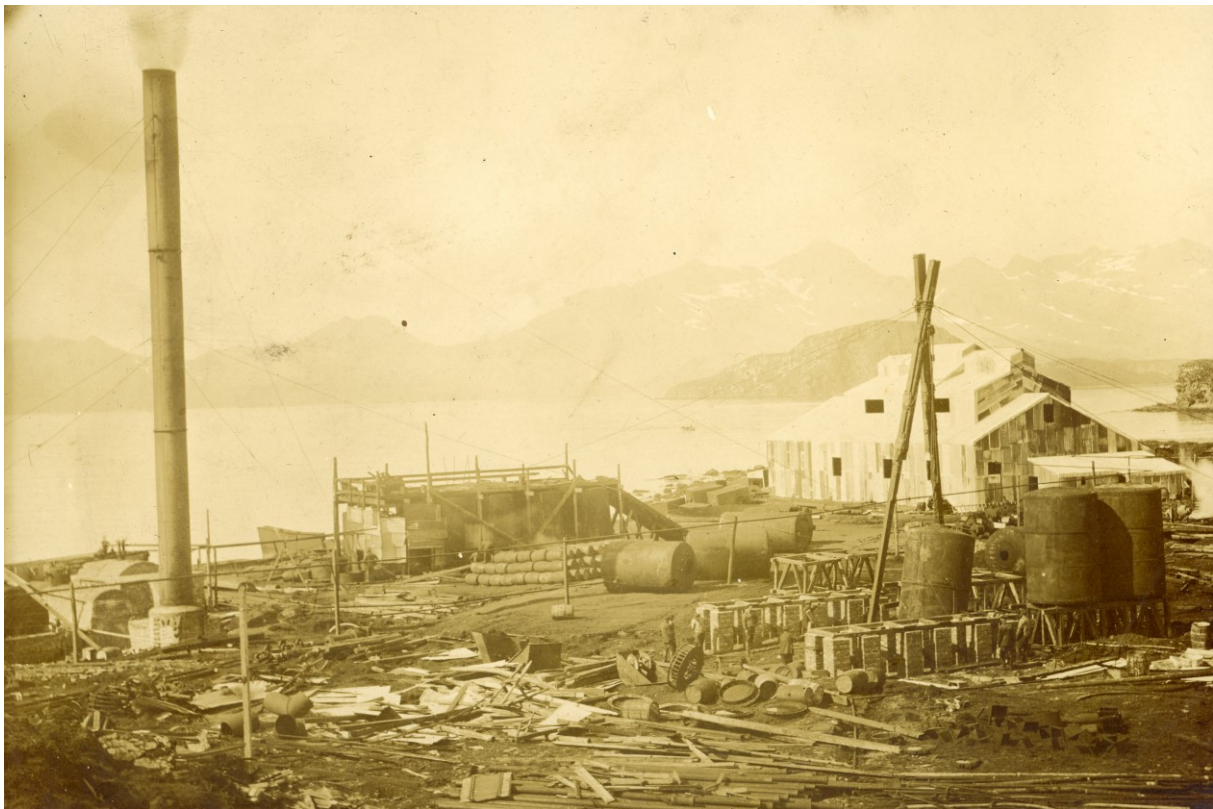
Fig 95. Construction work at Prince Olav Harbour. In the foreground the upper meat cookery is being assembled, and the lower meat cookery is not yet assembled. Below on the shoreline is the tongue cookery. Neither the lemming nor the flensing platforms are built. The photo has been published with the kind approval of the Kommendør Chr. Christensen's Hvalfangstmuseum. Norway.
