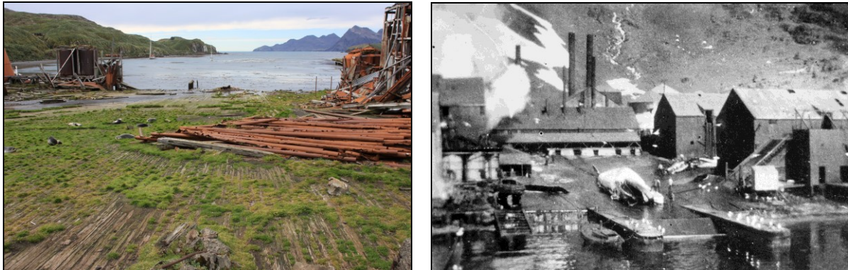
Fig 101 and 102. The wooden flensing plane at Prince Olav Harbour in 2009. Right: A whale has just been towed onto the flensing plane, and flensing of the blubber layer has commenced. In the front of the photo, the small motor boats the workers used to tow the whale from the buoy to the station are visible. To the right are the two meat cookeries (upper and lower), and the tongue cookery. Photo taken by Gustav Rossnes. LASHIPA 6/2009. Right: The photo has been published with the kind approval of the Kommendør Chr. Christensen's Hvalfangstmuseum. Norway.
