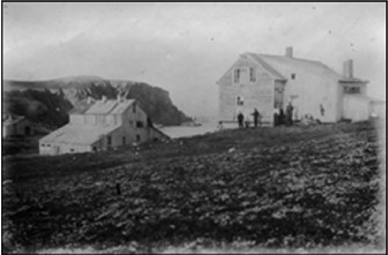
Fig 82. The accommodation house at Walrus Bay whaling station. The station only had one house that was used to accommodate all workers, which meant that skilled and un-skilled workers were not separated as was the custom in many whaling stations in the Antarctic. Behind it is the production area with the blubber cookery and the forge on the ridge beyond. 571
