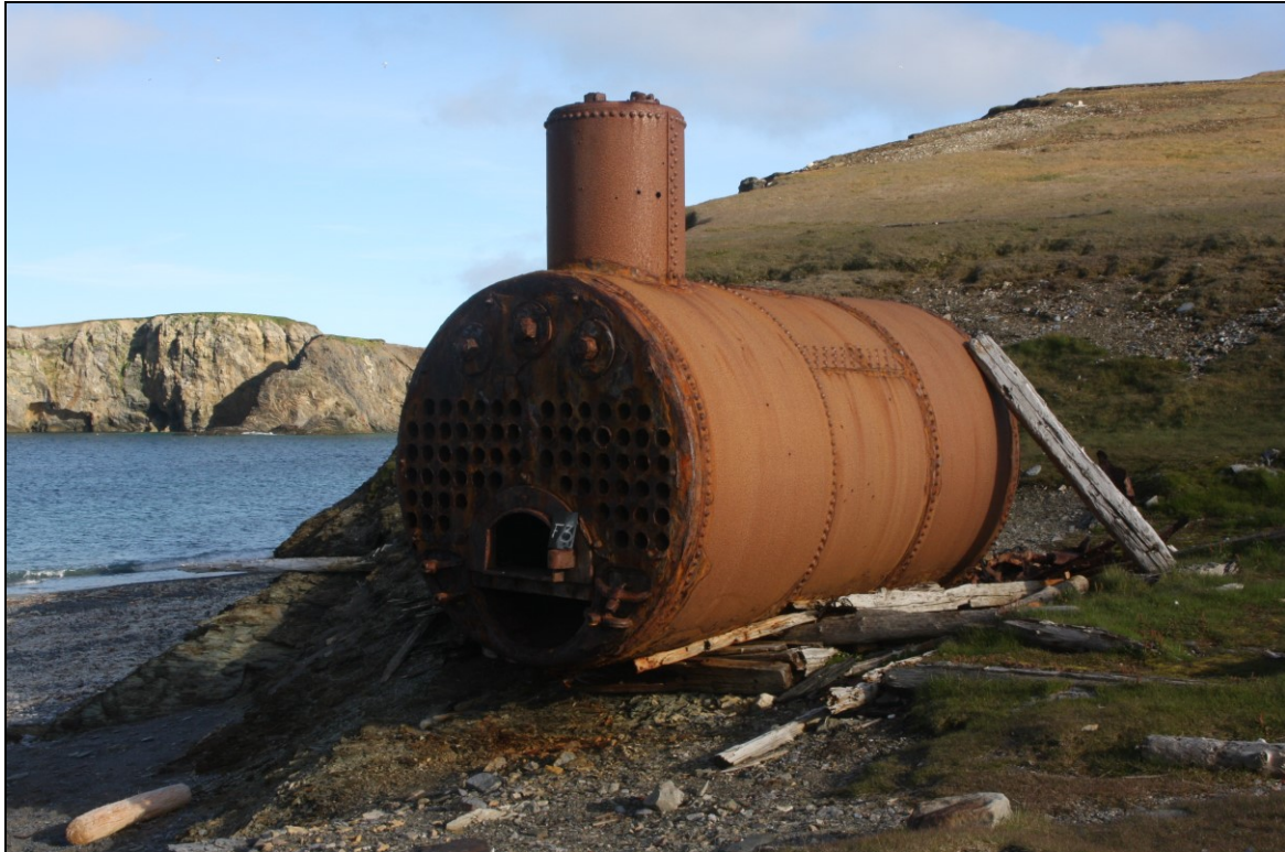
Fig 80. A steam boiler that still stands in situ at Walrus Bay. This boiler was used to generate the heat and pressurised steam that was necessary to run winches and cookers for processing raw material into liquid oil. Photo: G. Rossnes. LASHIPA 5/2008.
