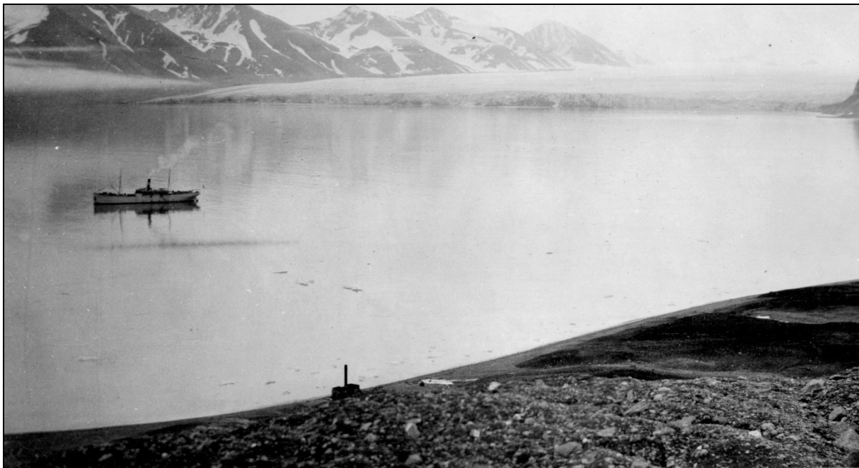
Fig 26. Land-based construction along the shores of Recherchefjorden on Spitsbergen. The photo was taken by an unknown employee of the Arctic Coal Company in 1913. The photo has been published with the kind permission of Michigan Technological University, USA.
