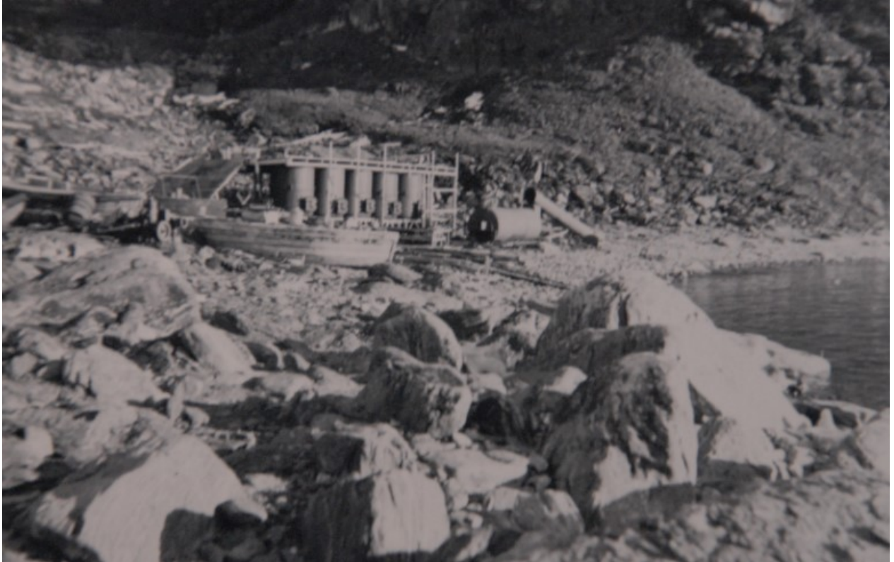
Fig 176. The remains of Signy Island whaling station during the 1940s. Today there are few remains of the whaling station, as much of it was removed during the building of the British Antarctic Survey research station. The tilting planes between the flensing and the elevated lemming platform are visible, as are the steam boiler and one of the barges that were used to transport blubber and water. The photo has been published with the kind approval of the estate of David Wynn-Williams.
