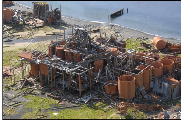
Fig 104 and 105. The design and internal layout of the blubber cookery at Prince Olav Harbour. Drawing by B.L. Basberg. LASHIPA 6/2009. Right: Overview over the blubber cookery. The cookers are located in the centre of the feature, and are surrounded by a large number of cooling/settling tanks. Photo: U.I. Gustafsson. LASHIPA 6/2009.
