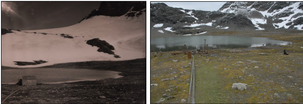
Fig 162 and 163. In 1923, Berntsen extended the local network at Signy Island by establishing a pump house next to a nearby glacial lake. This was connected to the beach by an iron pipe to secure a constant supply of freshwater. In the 1950s, the house was still in situ. Today, it has collapsed and is in a poor state. The photo on the left has been published with the kind approval of the archival services of the British Antarctic Survey. 1018 Right: Photo by U.I. Gustafsson. LASHIPA 8/2010.
