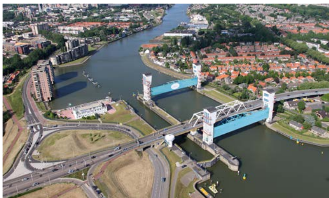
Figure 1: The Algera Complex [beeldbank.rws.nl].
