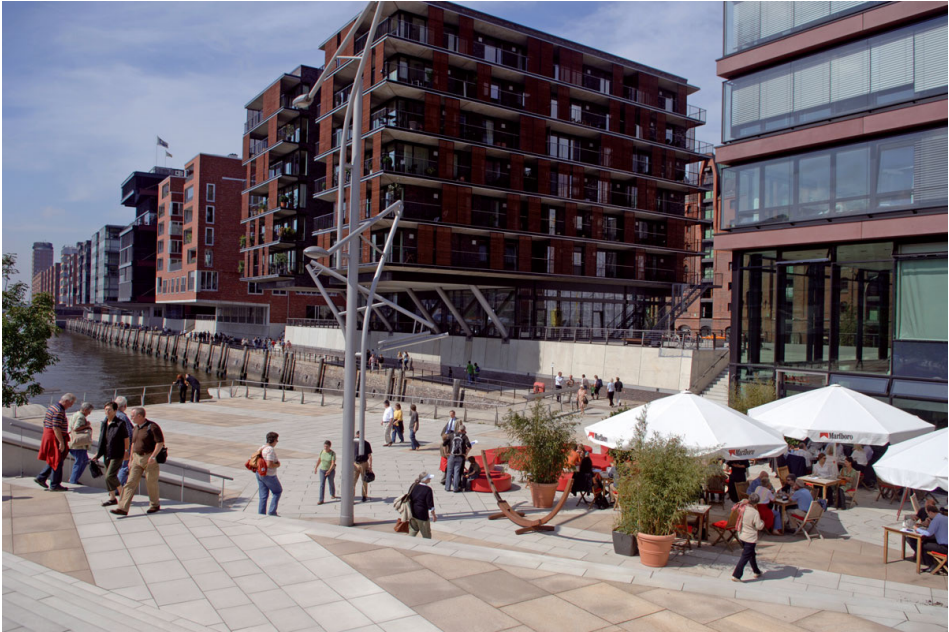
Figure 5.3: Basements of buildings, usual situation. Source: ELBE&FLUT/Thomas Happel.
