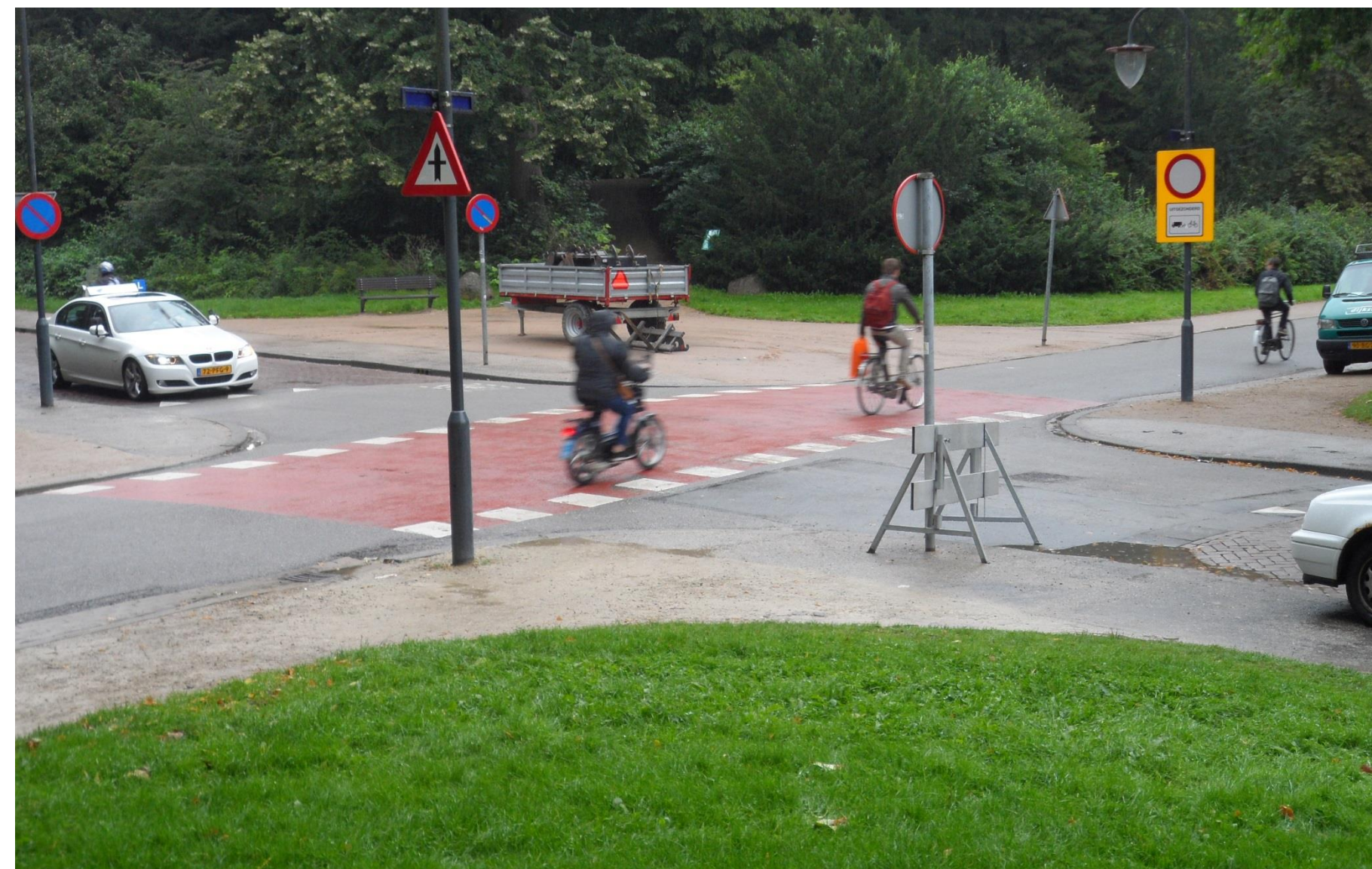
Figure 1: intersection with priority regulation (Kerklaan x Leliesingel in the Noorderplantsoen in Groningen, NL)
