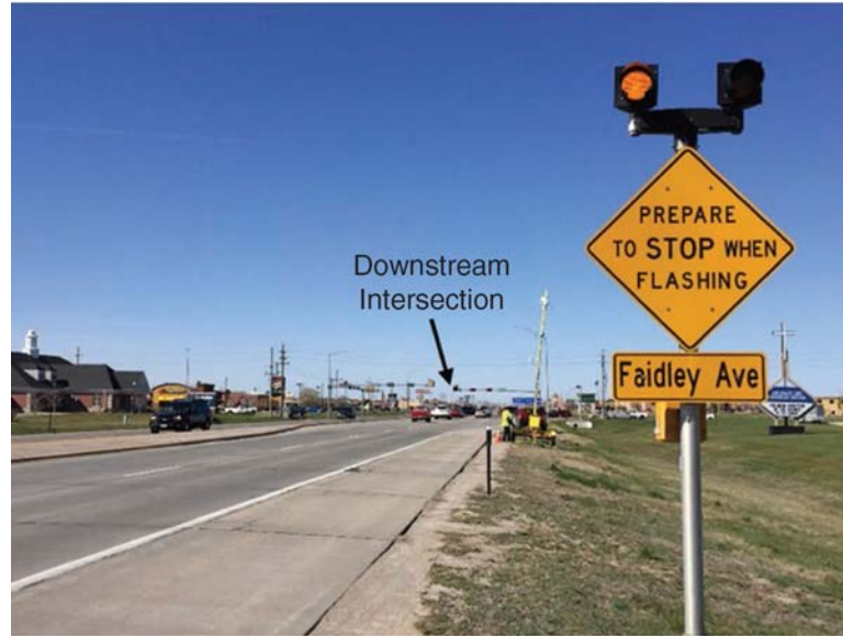
Figure 1. AWF and sign assembly, US-281, Grand Island, Nebraska.
