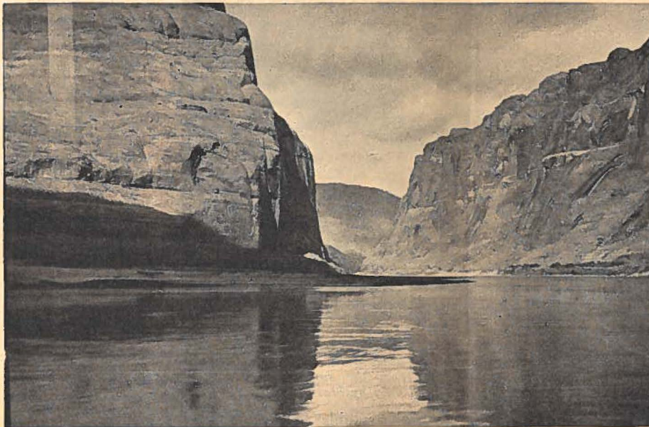
Glen Canyon dam site, on the Colorado, near Lees Ferry, Arizona, showing adequate abutments of a soft but massive sandstone.
