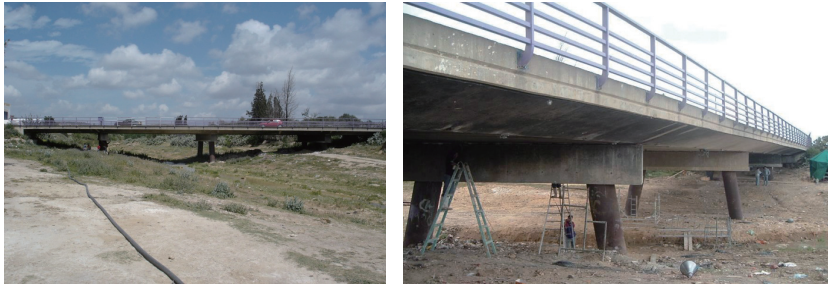
Fig. 1. Photographic views of the Béni Khiar bridge.
