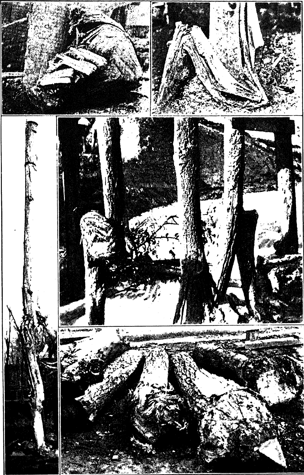
Damage of Timber Piles Caused by Overdriving
