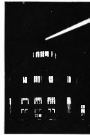
NIGHT VIEW OF AIRPORT OPERATIONS OFFICE WITH ROTATING BEACON ON TOP
