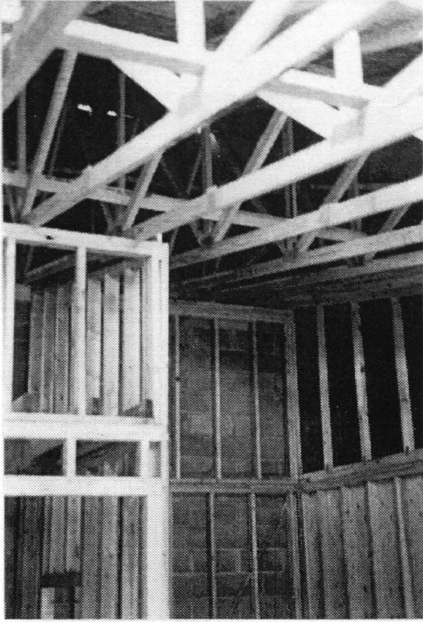
Installed Ceiling Trusses
