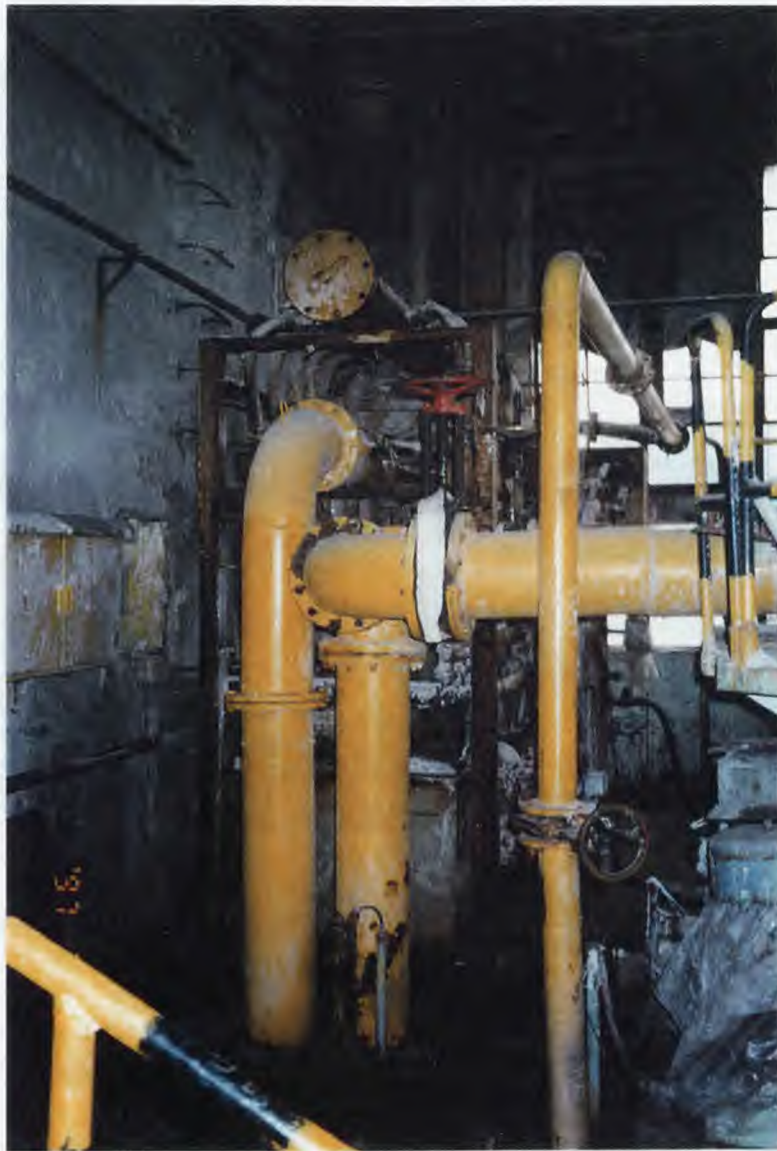
Photograph 10. Transporting the Slurry to the Paper Machine
