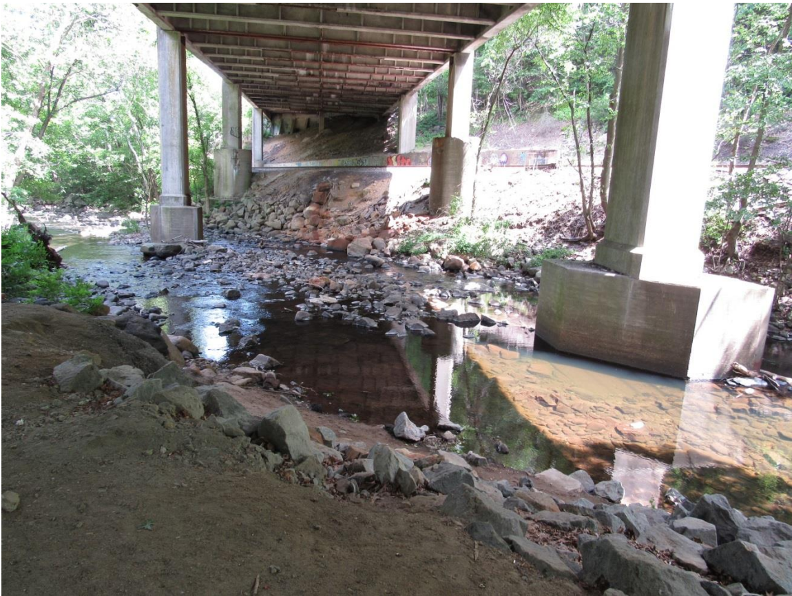
Figure E.25 Bridge # 1405-156 elevation, up-stream looking down-stream.
