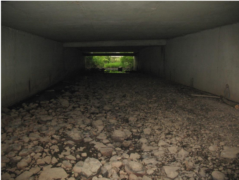
Figure E.1 Bridge # 0709-150 elevation, up-stream looking down-stream.
