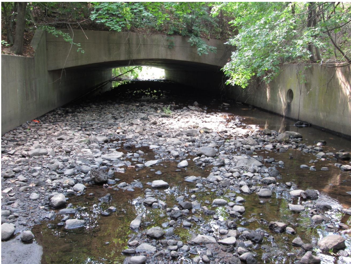
Figure E.10 Bridge # 1612-154 elevation, up-stream looking down-stream.
