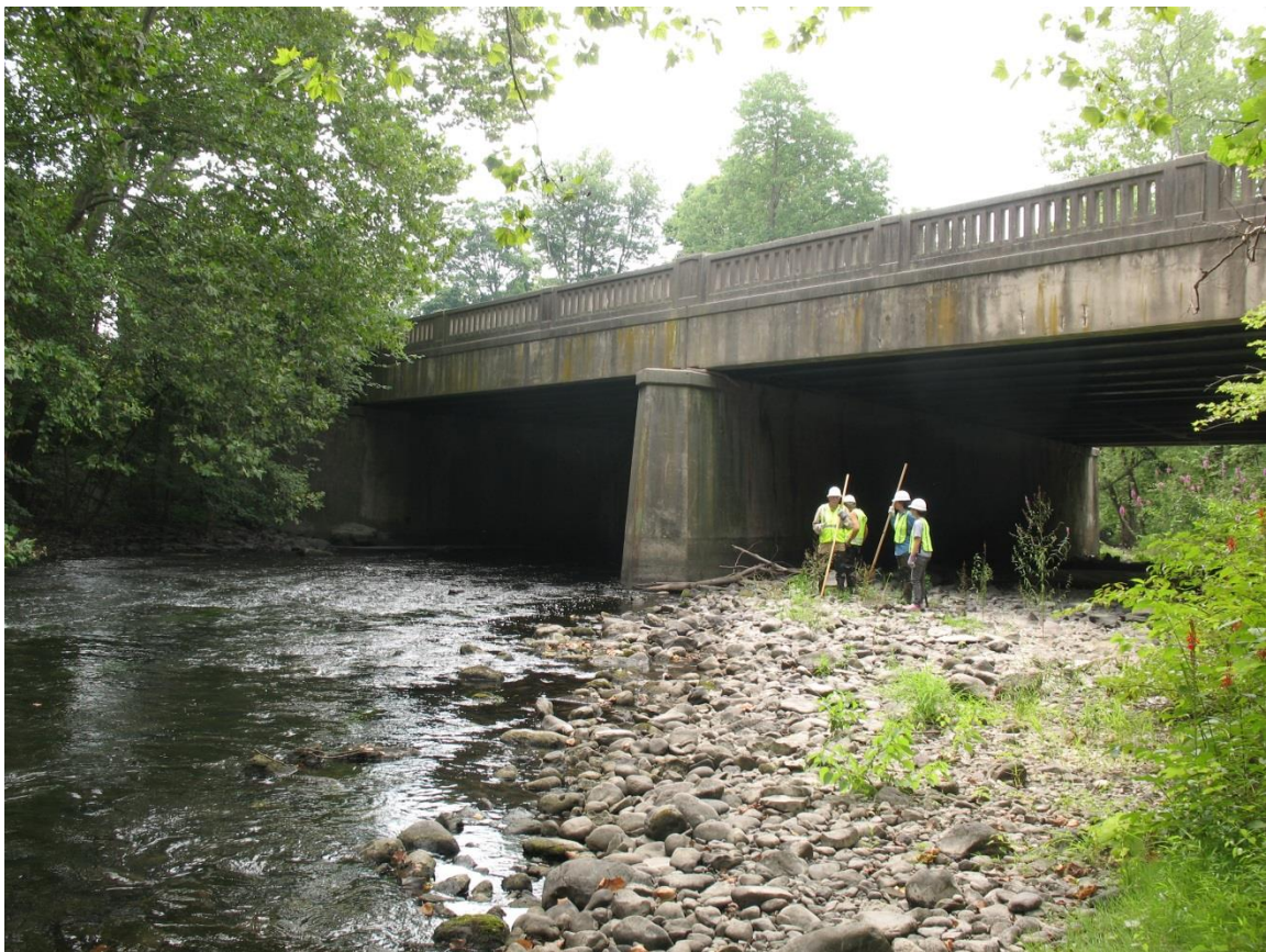
Figure E.31 Bridge # 2107-156 elevation, up-stream looking down-stream.
