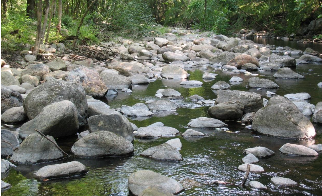
Figure E.23 Bridge # 1605-153 stream-bed sediments close-up.
