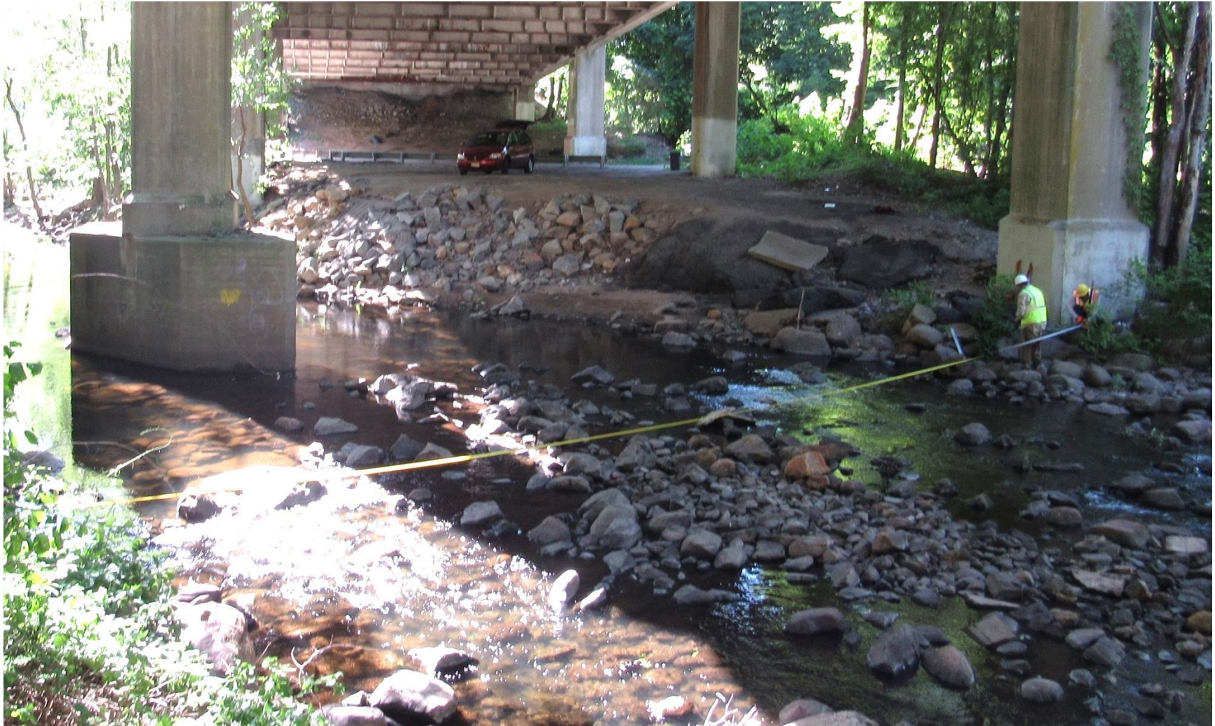
Figure 3.4 Wolman Pebble Count section installation, bridge # 1405-156.
