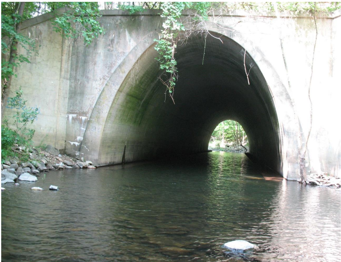
Figure E.22 Bridge # 1605-153 elevation, up-stream looking down-stream.
