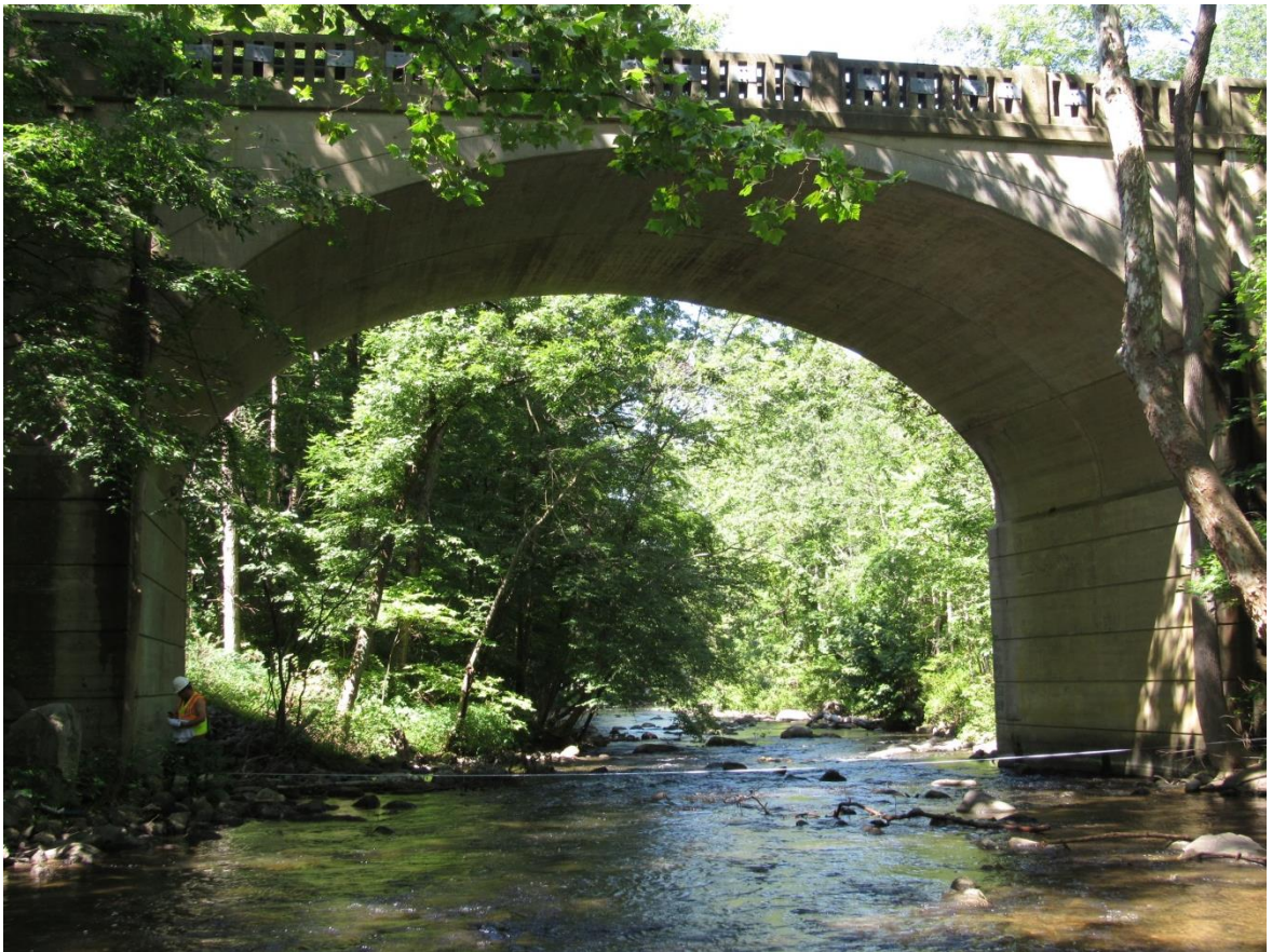
Figure E.34 Bridge # 2111-155 elevation, up-stream looking down-stream.
