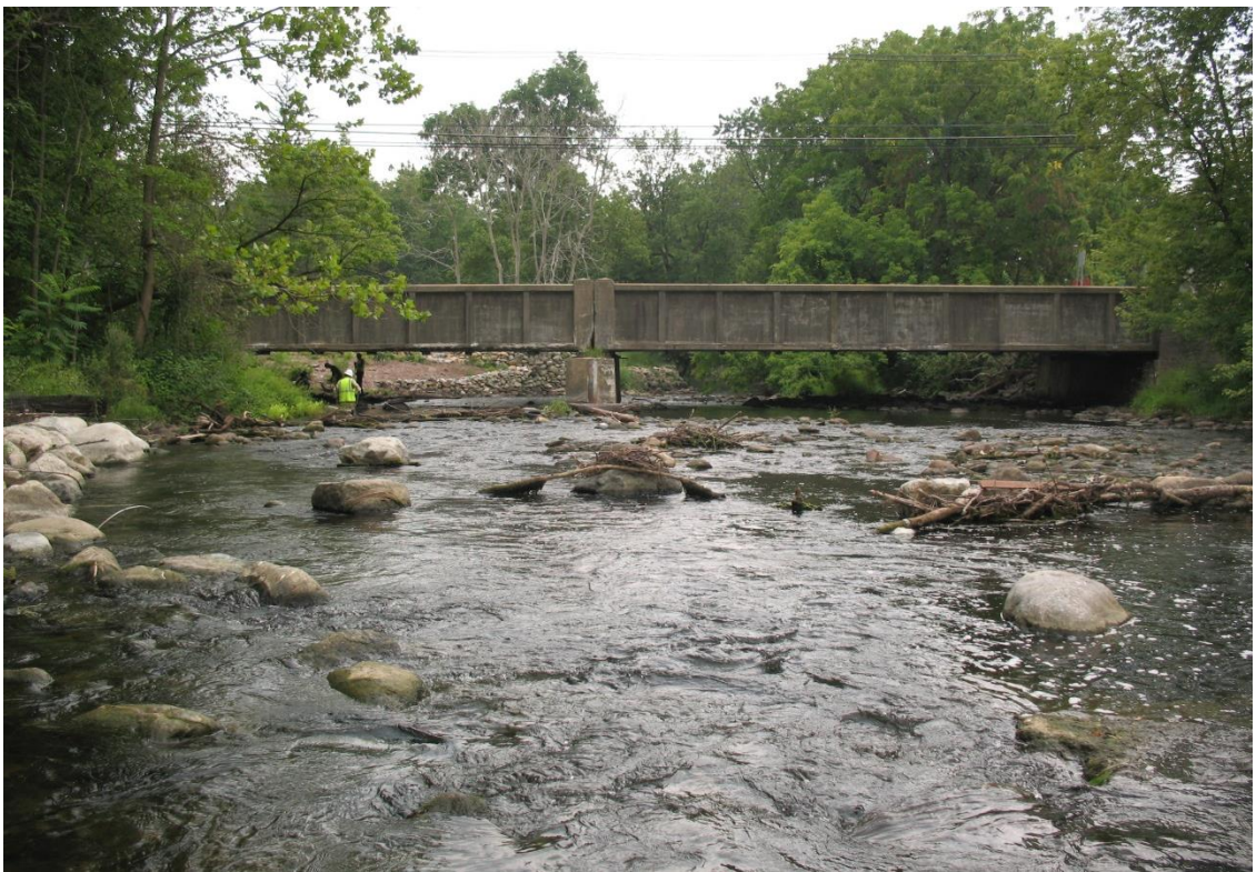
Figure E.13 Bridge # 2108-162 elevation, up-stream looking down-stream.
