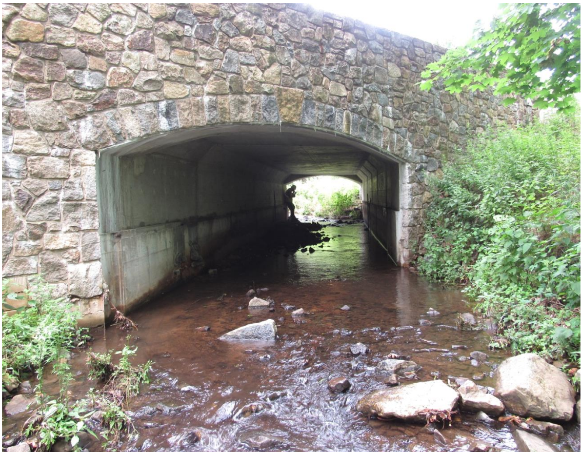
Figure E.4 Bridge # 1809-153 elevation, down-stream looking up-stream.
