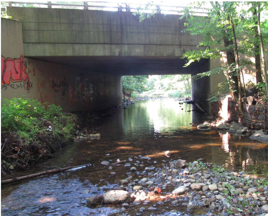
Figure E.7 Bridge # 0711-150 elevation, down-stream looking up-stream.
