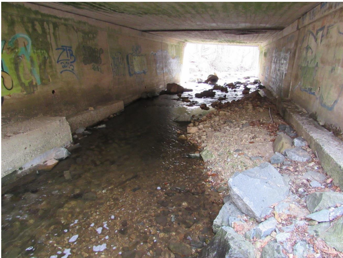
Figure E.19 Bridge # 1417-156 elevation, up-stream looking down-stream.
