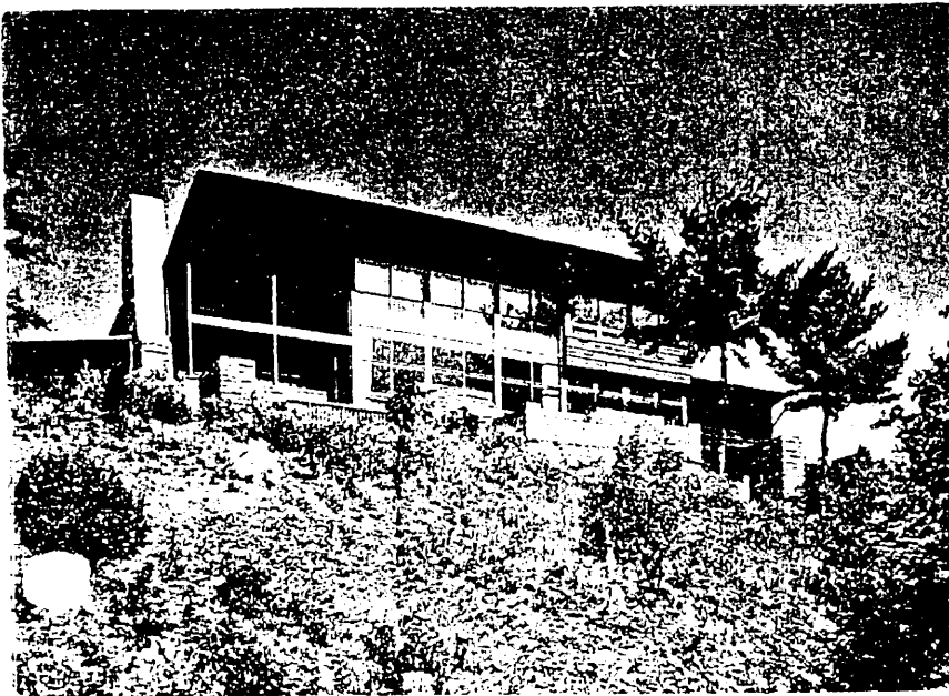
Figure 2.3 Exterior view from south-east
