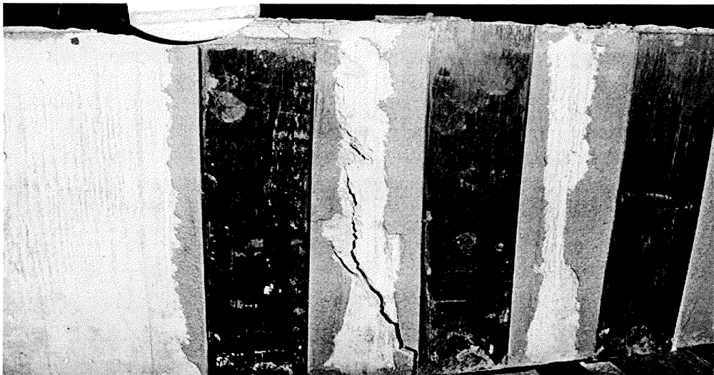
Figure 3.16 Failure of beam 2-3 with 90 degree aligned CFRP at right support
