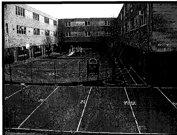
I.9 Fencing separates the inner-court renovated playground from the blacktop play area (foreground). The entrance gate is locked after school hours.
