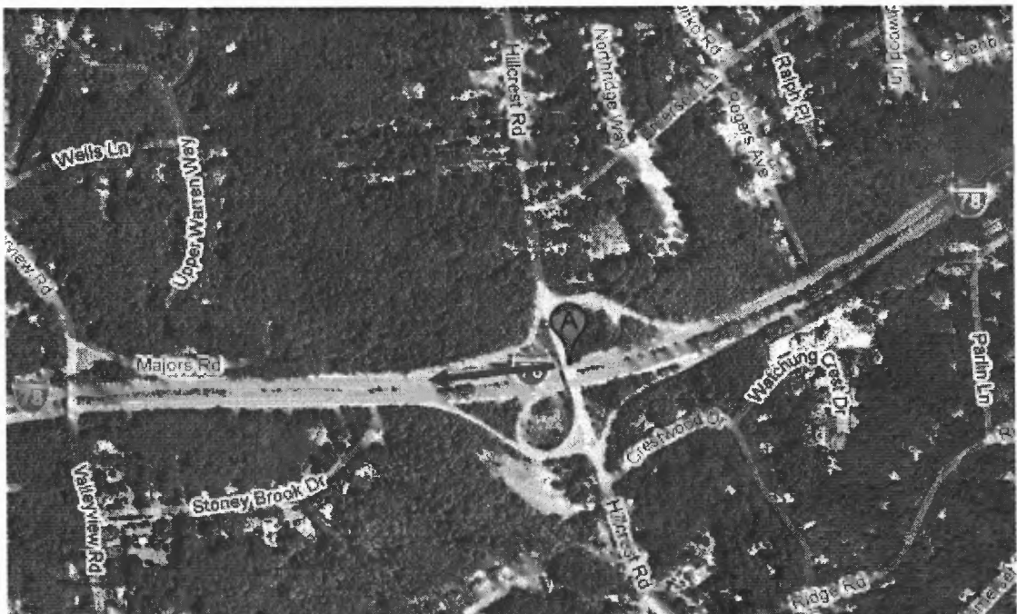
Figure 3.9 I-78 Road Structure and Geographic Location (Source: http://maps.google.com )
