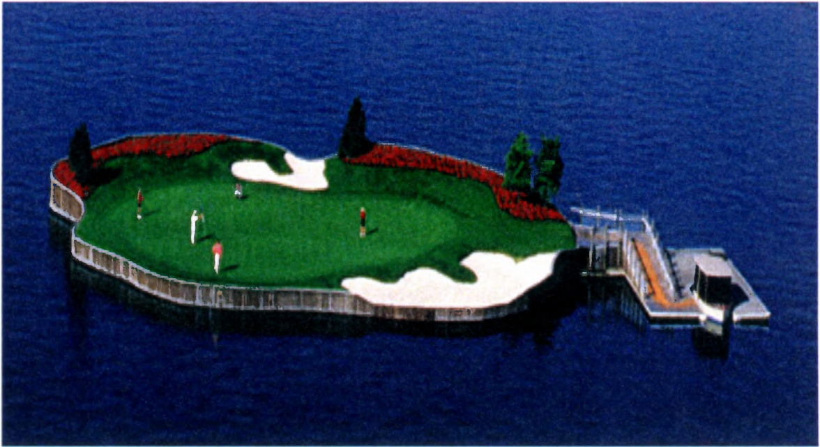
Figure 1.1 Fourteenth Green at Coeur d'Alene Country Club and Golf Resort in Idaho. The 15,000 ft 2 green is a man-made island that floats on an expandable polystyrene base, which is used to provide structural support and integrity while also providing the necessary buoyancy. Photo from Hagadone Hospitality, 2001.
