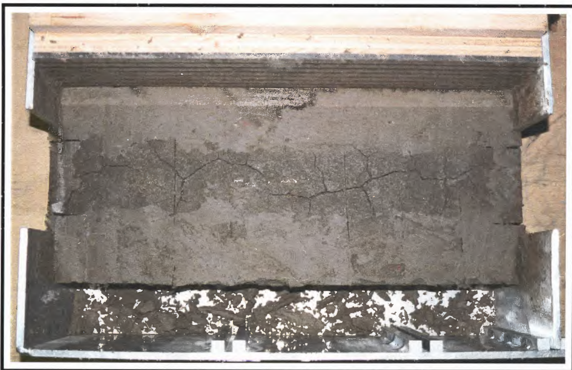
Photograph A-12. Shrinkages cracks were apparent in the soils 1 in. above the fracture. The cracks are approximately 1 to 2 mm wide.
