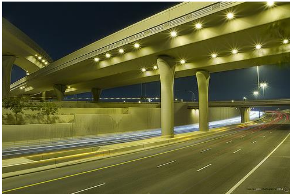
Figure 2.63 Side view of the bridge.
