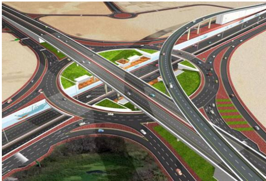
Figure 2.62 Aerial Photo of the bridge.
