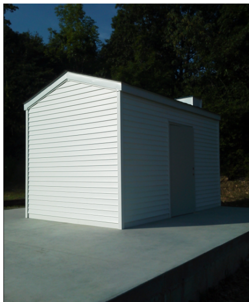
Figure 5.5 Concrete Slab With Electronics Shed
