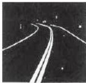
Figure 2.3 (a) Pavement markings with reflective beads.
