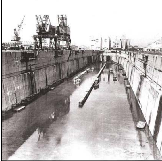
Figure 6.9 Bayonne Port Drydock. 1962. This facility, part of the peninsula pictured in Figure 6.8 removed ships from the water for maintenance and repairs.
