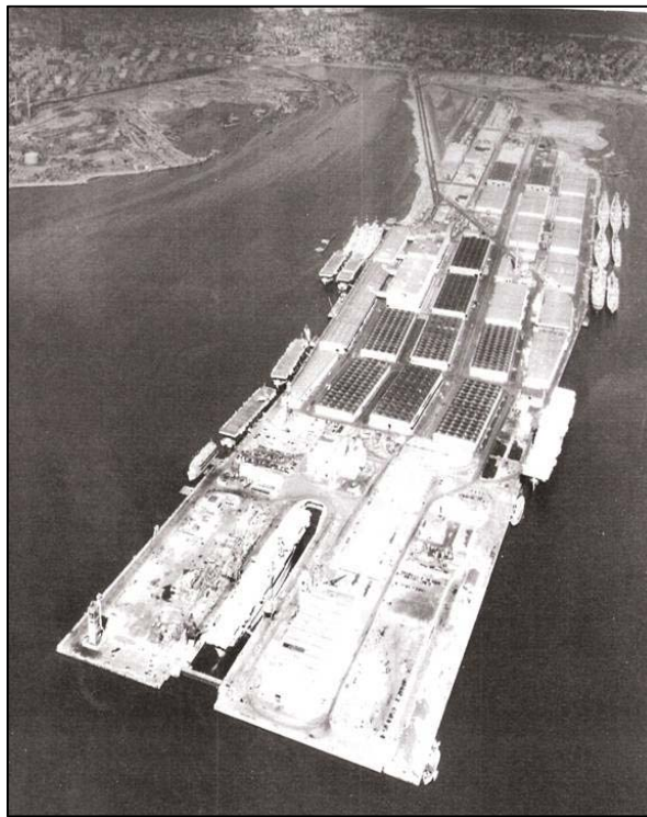
Figure 6.8 US Naval Supply Center, Bayonne. 1975. The peninsula pictured was constructed by the US Navy from dredged material and extended from the Bayonne waterfront into the Upper New York Bay.
