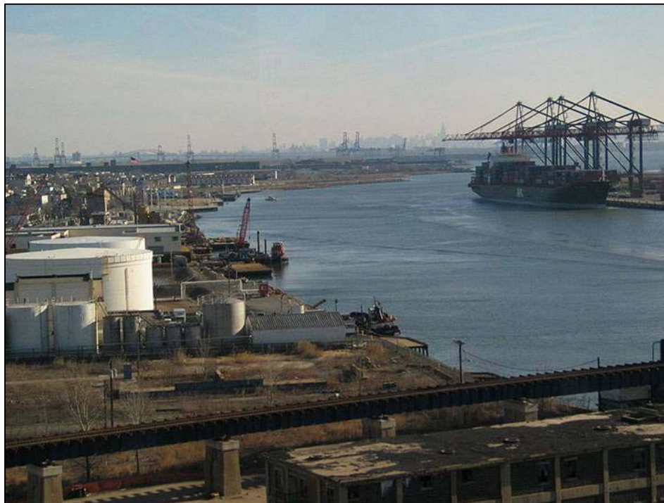
Figure 12.2 City of Elizabeth Waterfront, the Arthur Kill, and the Howland Hook Marine Terminal (from left to right). 2006. Photograph. Elizabeth-Port Authority Marine Terminal is in the background.
