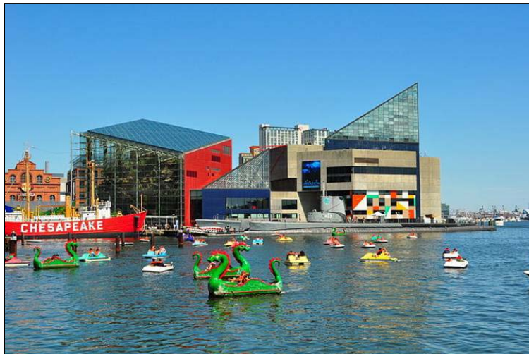
Figure 2.8 Baltimore National Aquarium. 2010. Photograph. The photo shows new uses (aquarium, recreation, retail) at a former port-abandoned waterfront.
