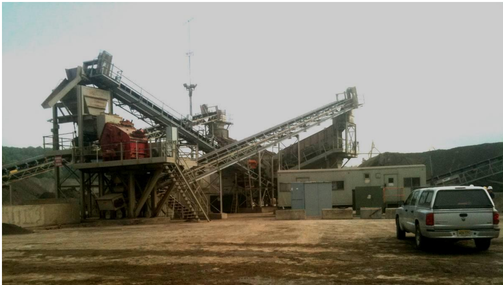
Figure 3.1 Weldon Materials crushing facilities, New Jersey.
