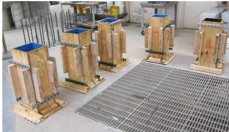
Figure 3.11 Plywood forms.
