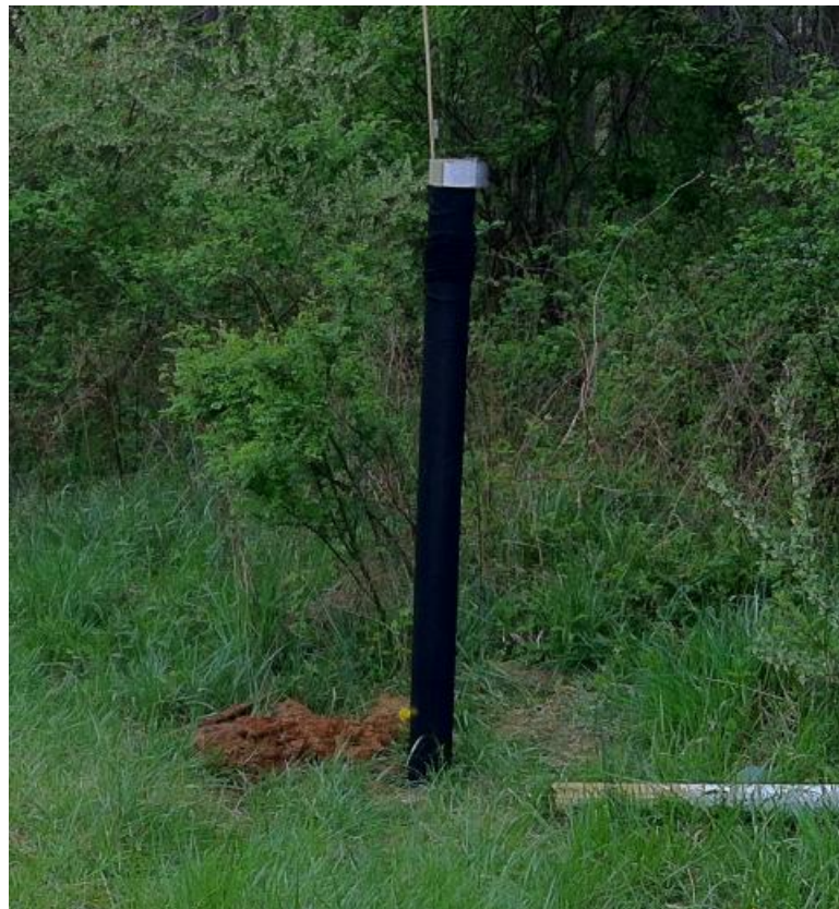
Figure 2.5 Perforated four (4) inch pipe covered by black filter sock.
