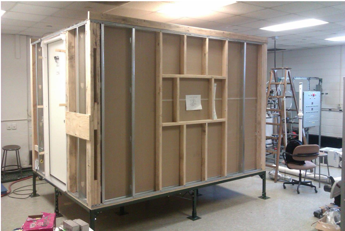
Figure 4.2 Actually experiment system of A/C chamber.
