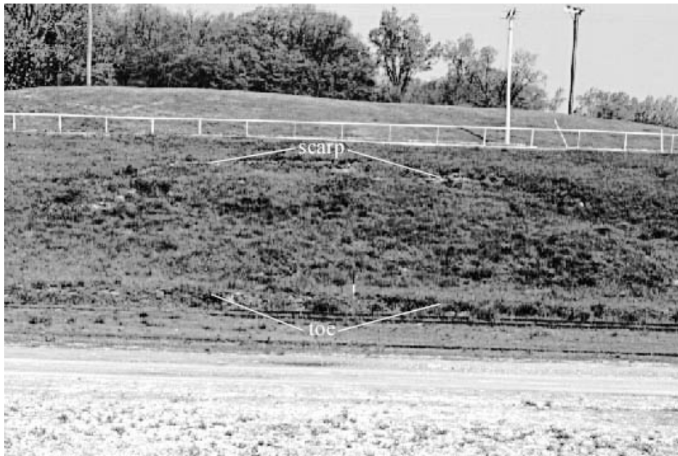
FIGURE 11. An earth flow at the U.S. Army underground storage facility in the south end of Atchison, Kansas (SW SE sec. 7, T. 6 S., R. 21 E.).
