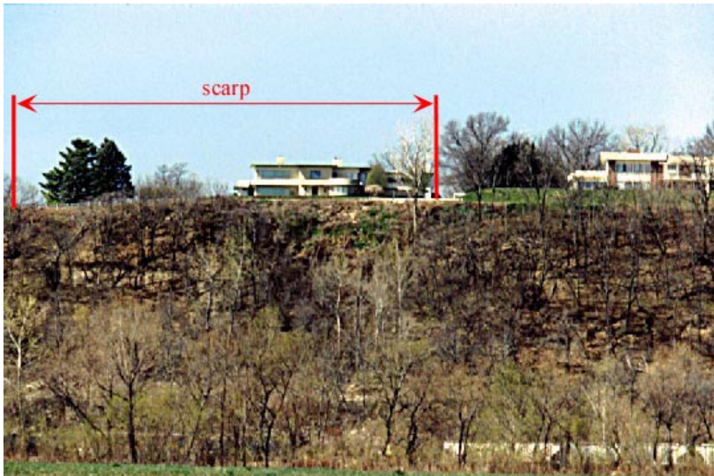
FIGURE 8. A recent landslide along Riverview Drive south of downtown Atchison (SW NE sec. 7, T. 6 S., R. 21 E.). The scarp (the surface break at the top of the landslide) is along the road at the top of the hill, and the toe (where material piles up at the bottom of the landslide) is at the base of the slope. The houses in the photograph are set back from the top of the hill and are not currently involved in the landslide.
