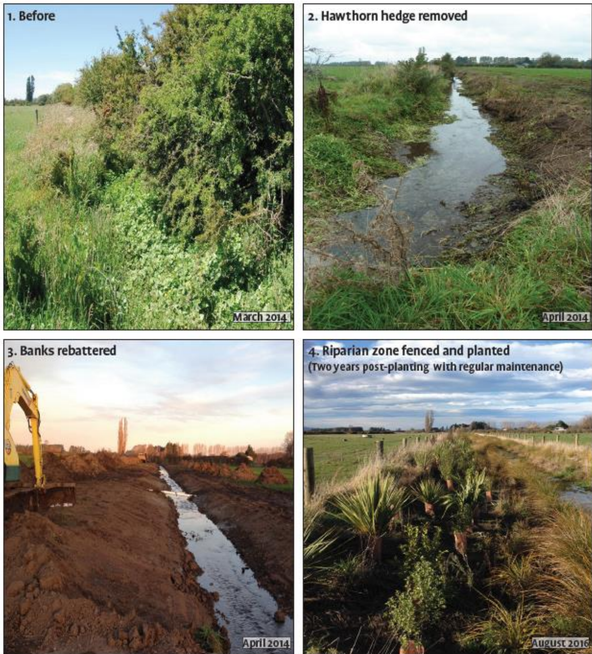
Figure 4-15 Example of Canterbury Waterway Rehabilitation Experiment (CAREX) Rehabilitation (Febria et al., 2018)
