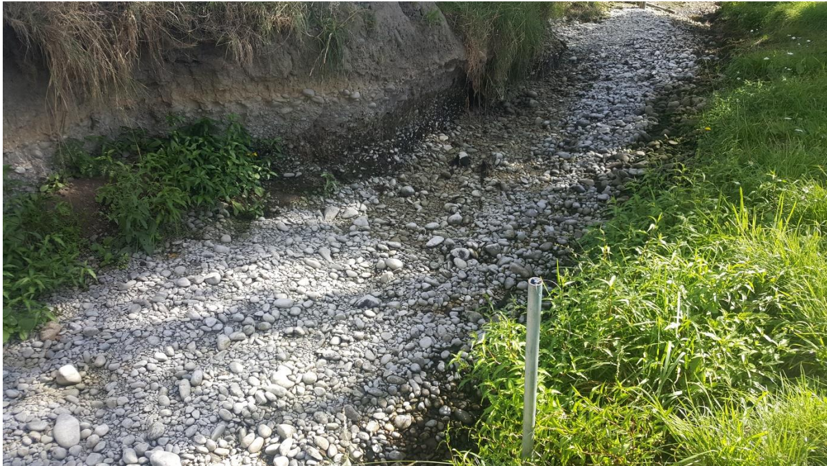
Figure 3-4 Windermere Drain at Lower Beach Road on 18 February 2018
