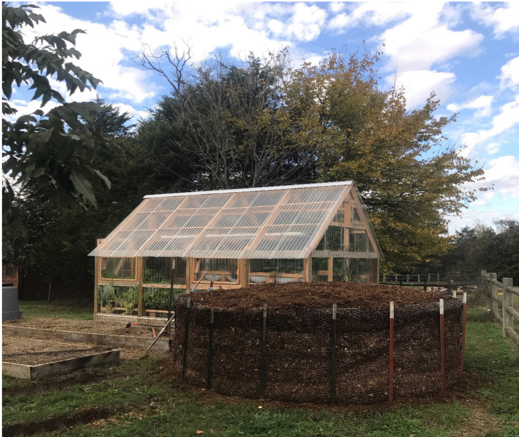
Fig. 1. Greenhouse structure with horse manure compost heater and raised garden beds for transplanting larger plants.
