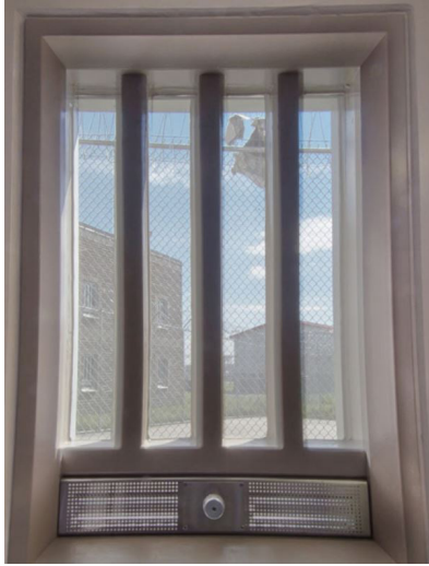
Figure 02-03-08. Window in maximum security cell, Collins Bay Institution, Canada
