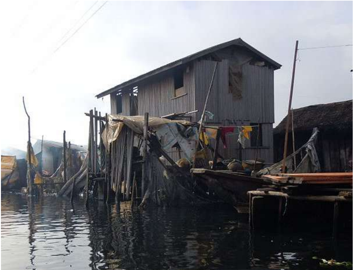
FIGURE 2.05 Typical multi-storey construction in Makoko
