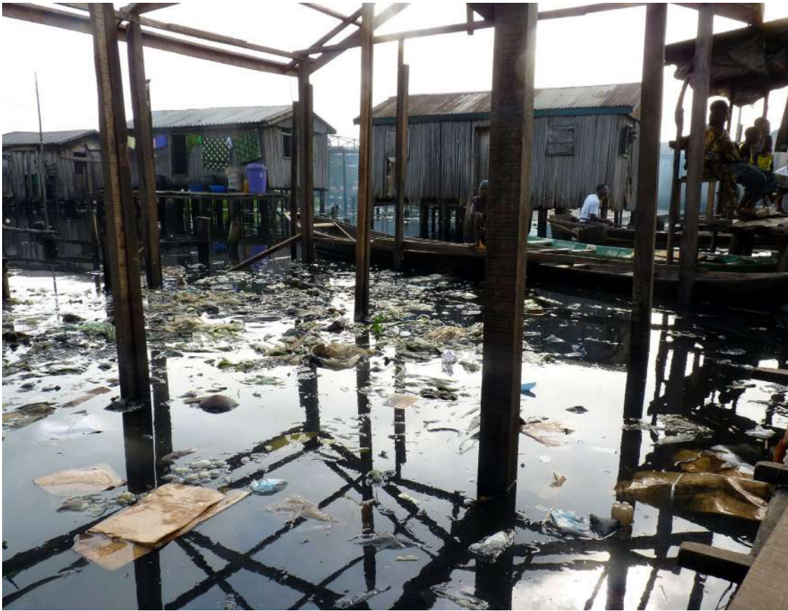
FIGURE 6.02 Typical flood conditions in Makoko
