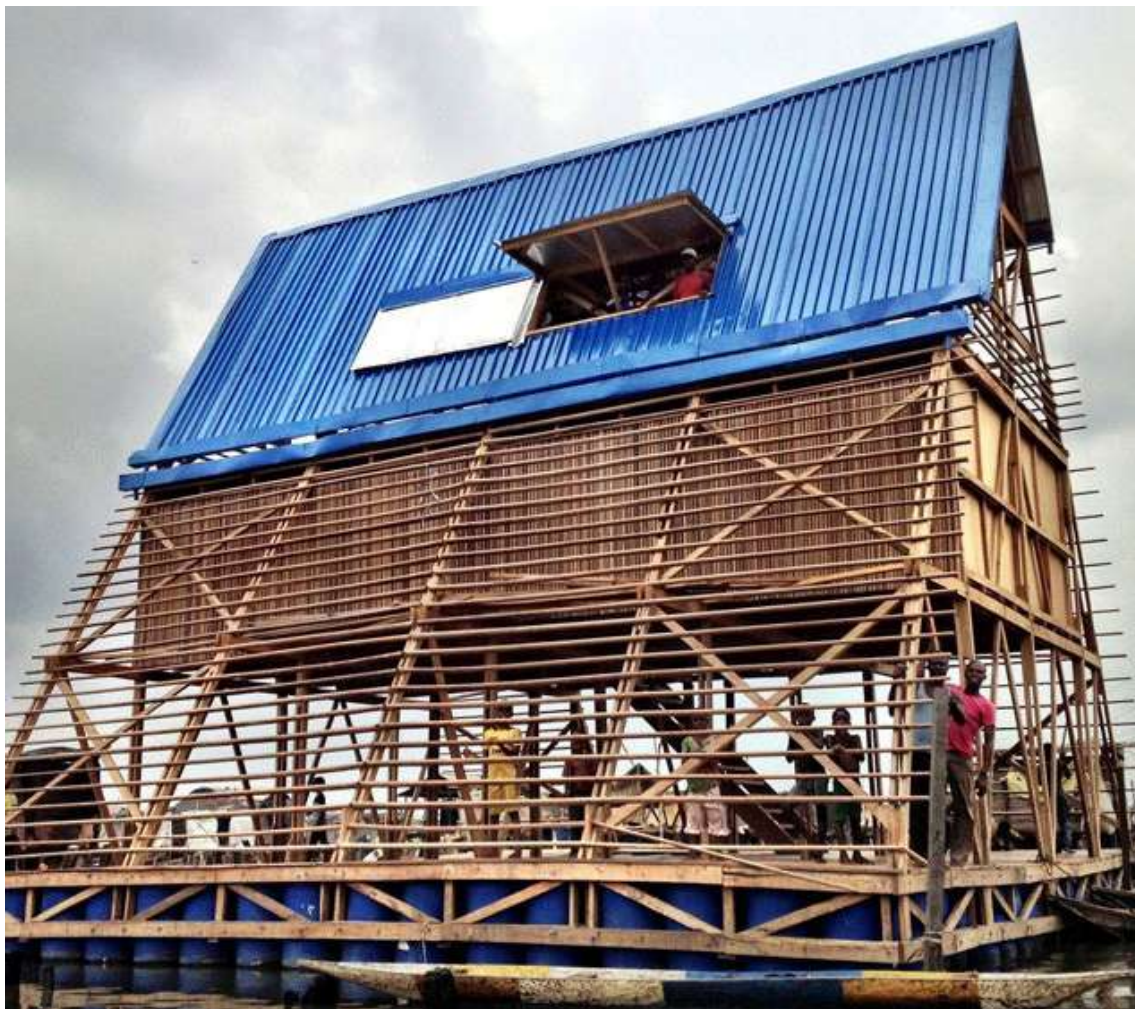
FIGURE 4.02 Makoko floating school A-frame structure by Kunle Adeyemi of NLE
