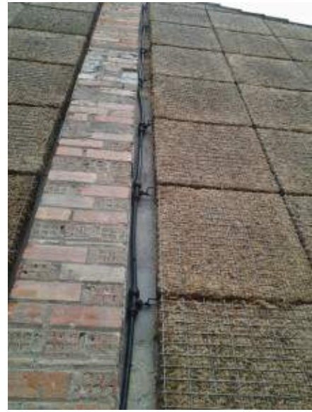
Figure 78.. Detail of automated irrigation system (Source: www.alijardin.es )
