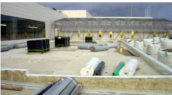
Figure 33: Protection material , draining element and filter sheet area
