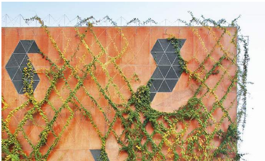
Figure 117. Green Facade in FECSA –ENDESA ,Barcelona
