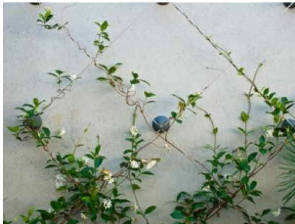
Figure 47 Figure. Braided cable system.
