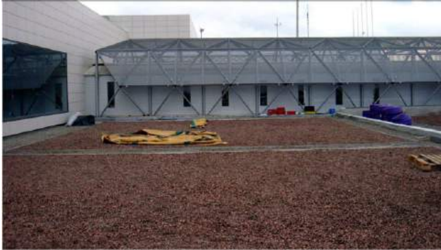
Figure 35 :the roof are with the substrate application
