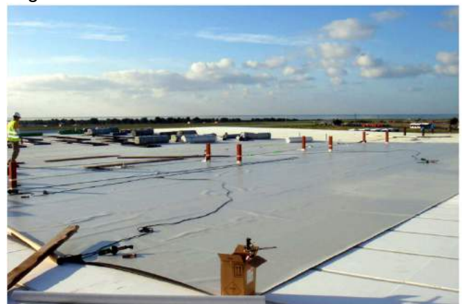
Figure 34 : Preliminary work on the roof (source : zinco-greenroof.com)
