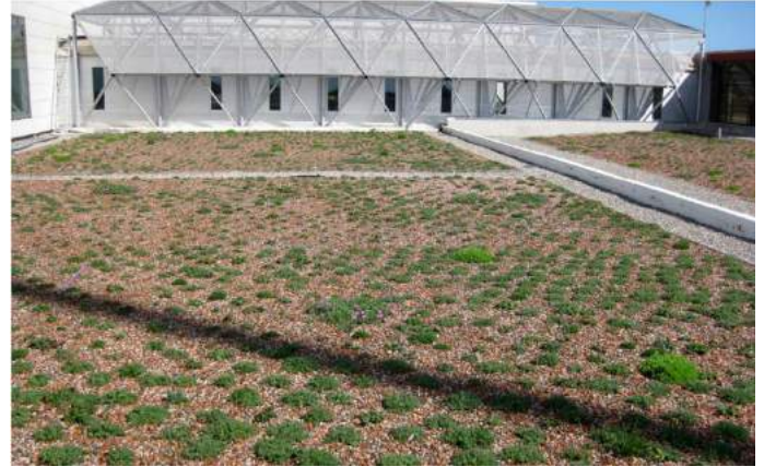
Figure 36:the roof area after a few months
