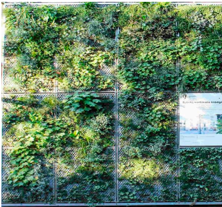
Figure 52.External Green facade with module lattice
