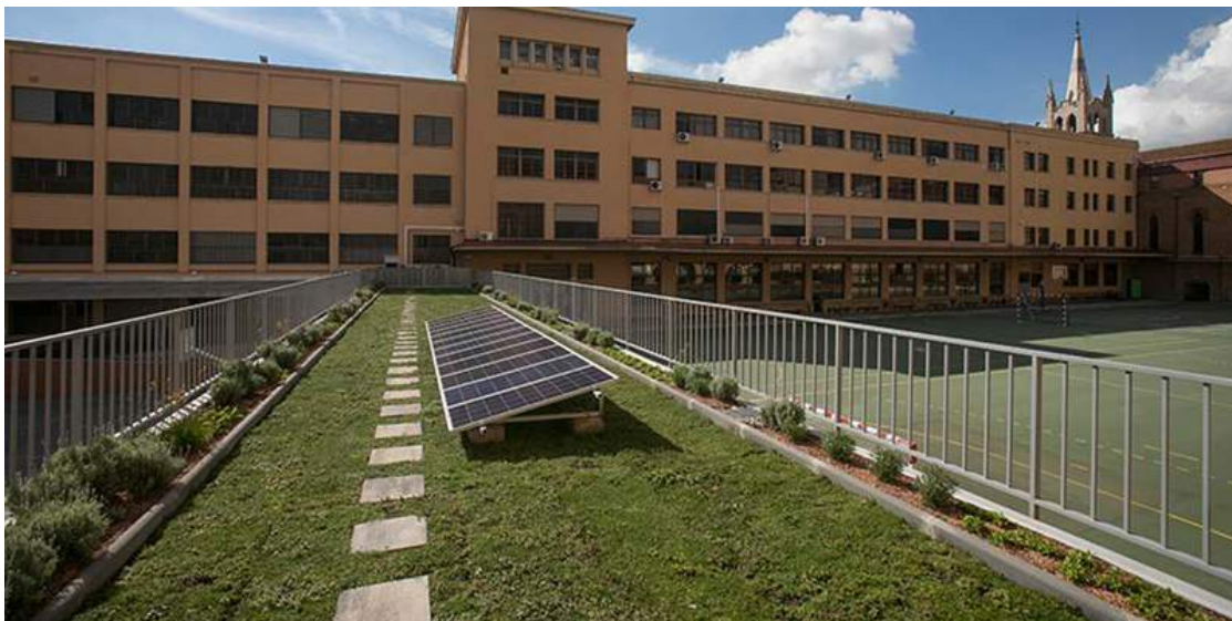
Case 3 Figure 108. Extensive green Roof Barcelona (source:construible.es)
