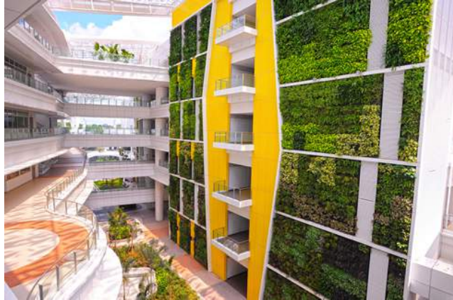
Figure 60 VGM modules allow the creation of instant green walls on both free standing walls and on building facades
