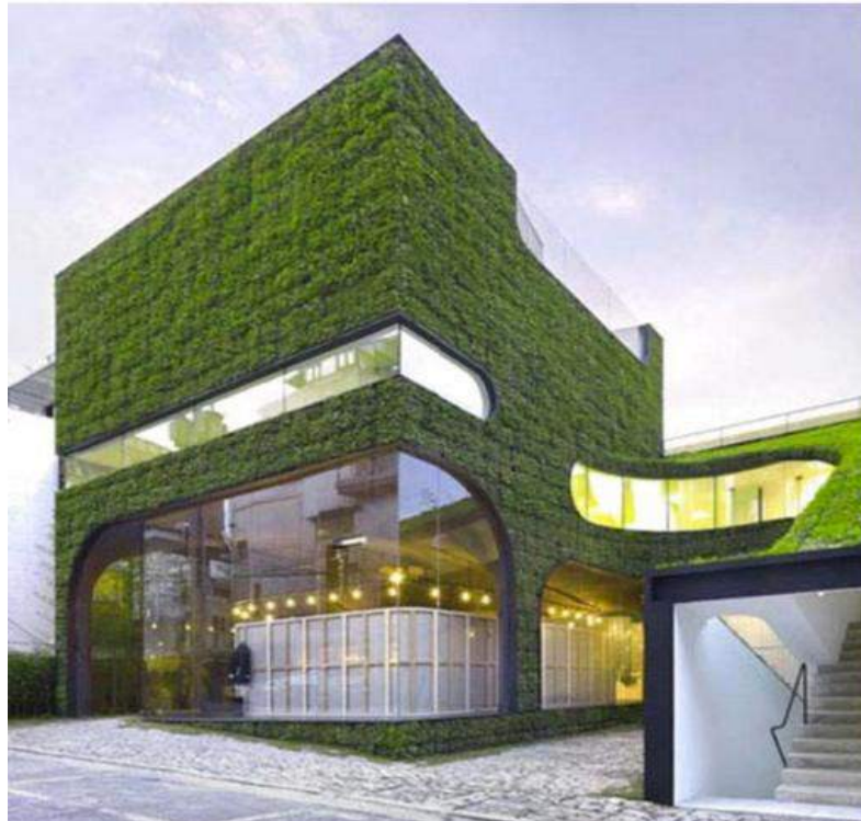
Figure 73. Shop design by Minsuk Cho Architect
