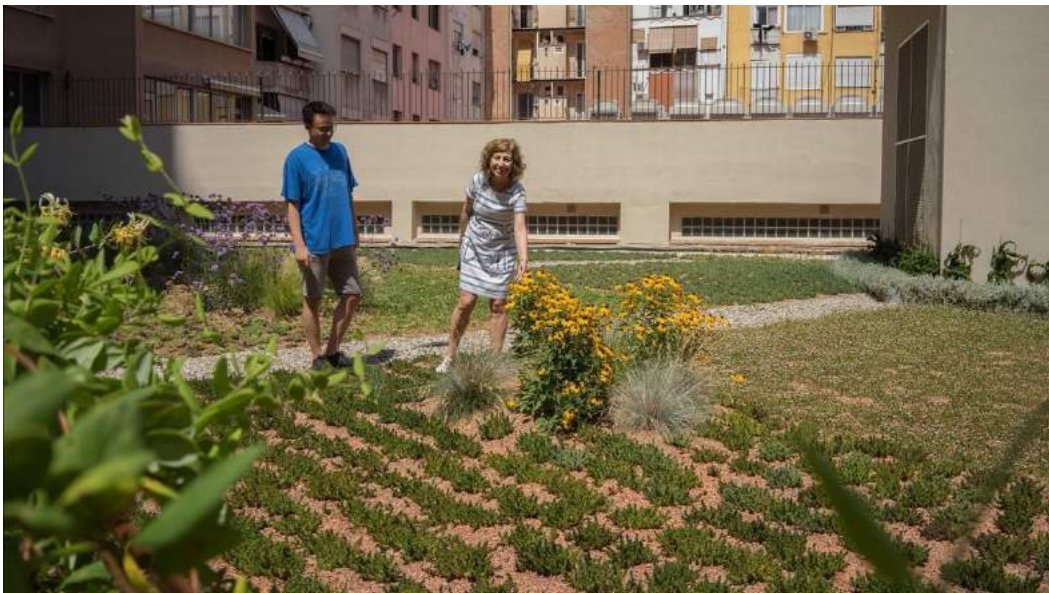
Figure 110: Private green roof building Aragon estate with Casanova, Barcelona
