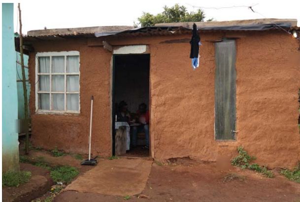
Figure 1: Backyard-bedroom studios, exterior view
