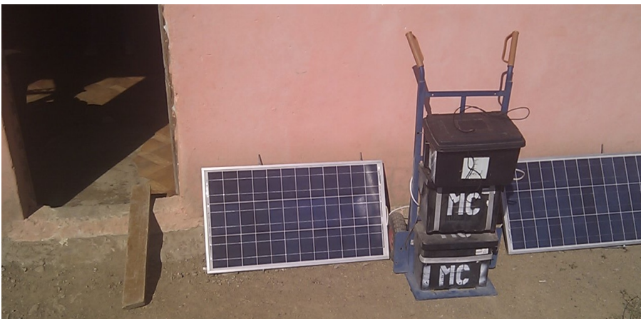
Figure 5: Plank over the door frame of the office at Ngcobo to guide Station (V2)
