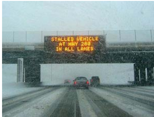
Figure 1: Variable Message Signs[24]
