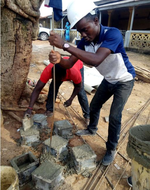
Plate II: Compacting of green concrete in layers
