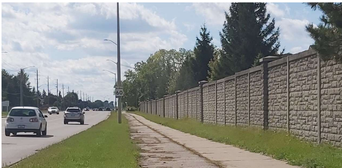
Figure 1-1: Example of a sound wall reducing traffic noise from entering residential area.
