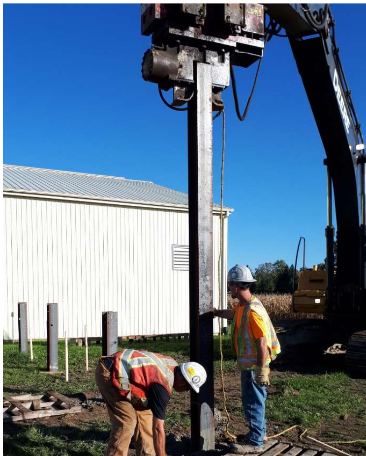
Figure 3-8: Vibratory driving of the steel piles.
