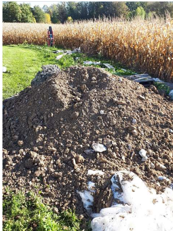
Figure 3-10: Soil and concrete waste from drilled shaft installation.
