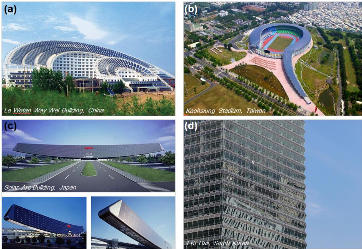
Fig.2. Representative BIPV buildings
