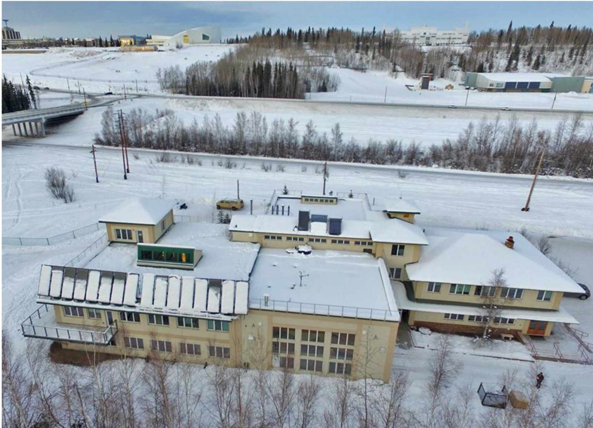
Figure 2.1. CCHRC's Research and Testing Facility. The original building (the right side of the photo) was built in 2006; the addition on the left was completed in 2012. The heat pump heats the section on the far right end of the photo.
