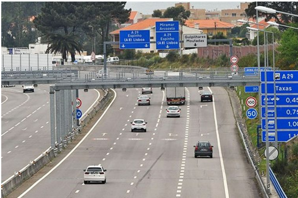
Figure 2.2: Portuguese tolls that use RFID for vehicle identification 2 .
