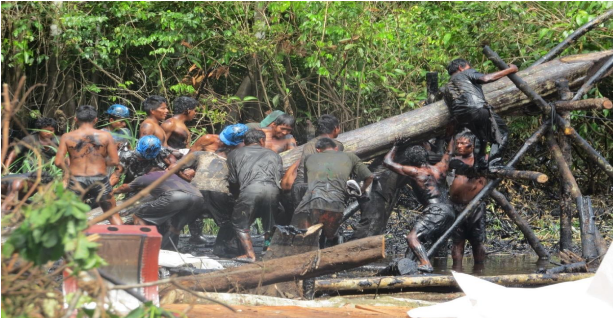
Photograph 7.5: Cocama residents inserting or removing one of the large wooden timbers that supports the pipeline.
