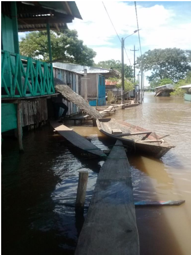
Photograph 6.8: Duckboards enable the community to move around during the annual flooding.
